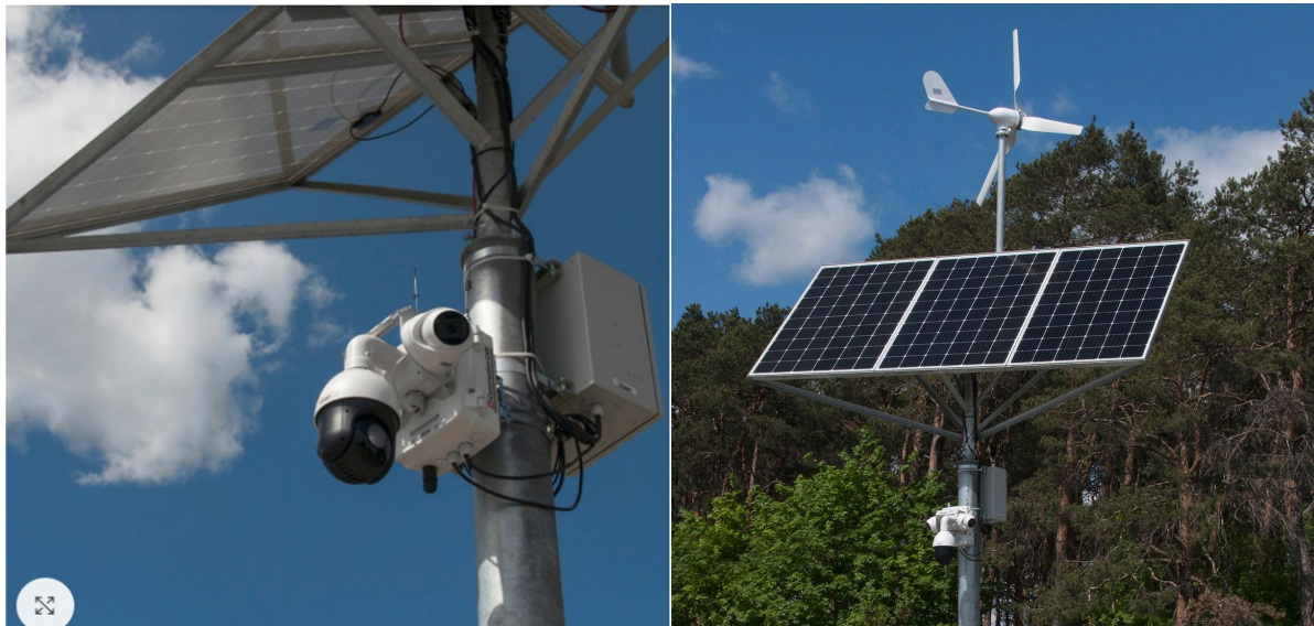
Figure 5 – Professional all-year solar power system for CCTV cameras
